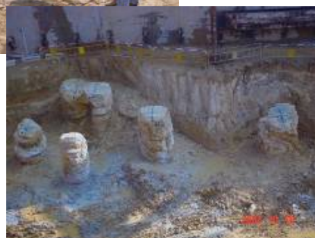
Trial Jet Grouting
