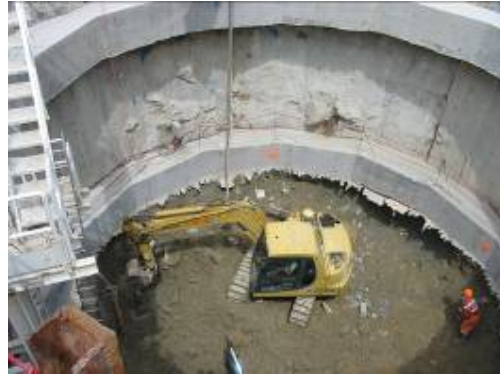
Ring beams are casted during the progress of the bulk excavation.
