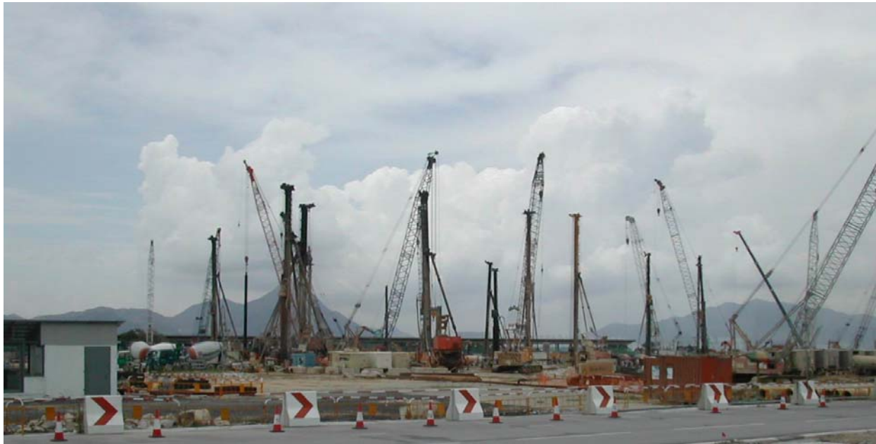
The IEC site during the piling works.
