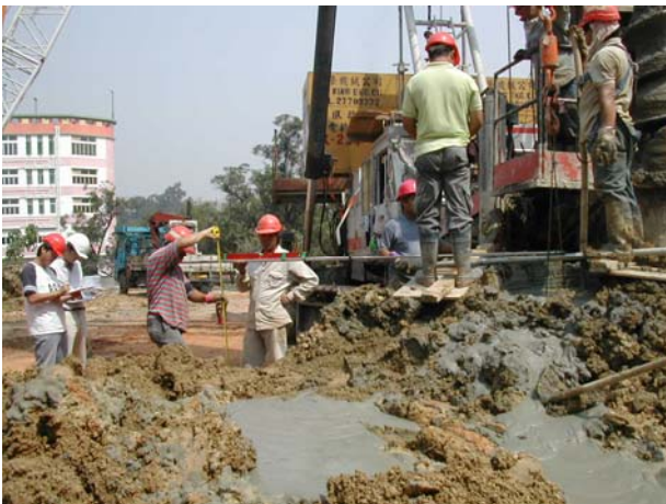
Check As-Built Pile Position
