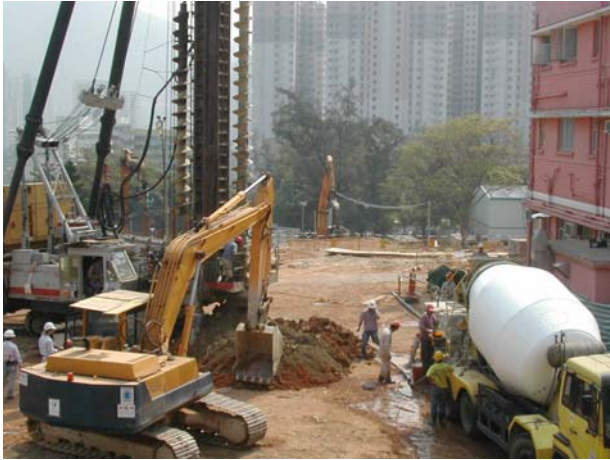
Drilling and Grouting of Pile
