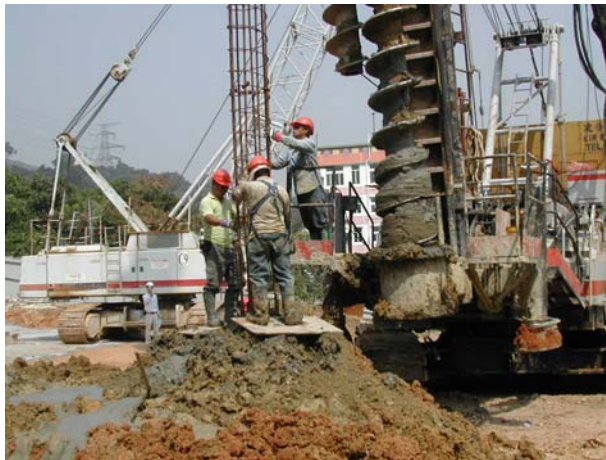
Steel Cage Installation
